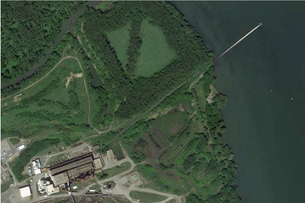
Figure 2-1 Aerial View of the Greenidge Generating Station (lower left) showing Unit 4 intake conduit extending to Seneca Lake.
