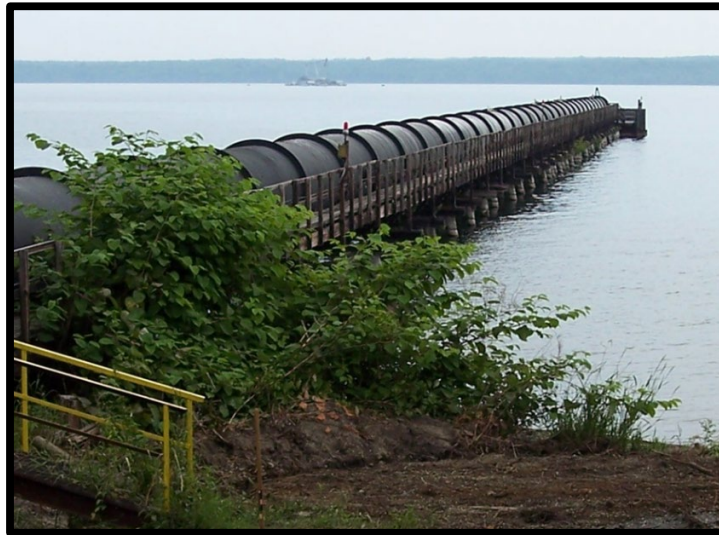
Figure 1.2: Unit 4 withdrawal conduit extending from the west shore of Seneca Lake.
