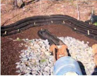
Figure 5.25 Pipe Outlet Sediment Trap: ST-I
