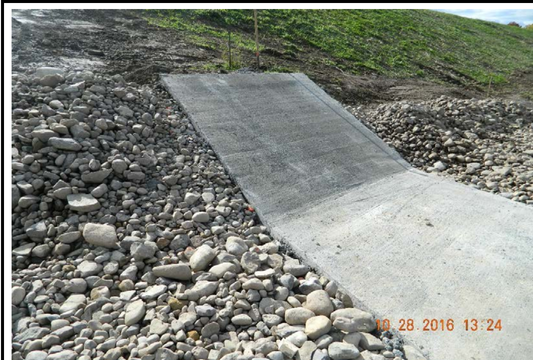
Photo 60: Concrete lined channel, looking southwest (10/28/16)
