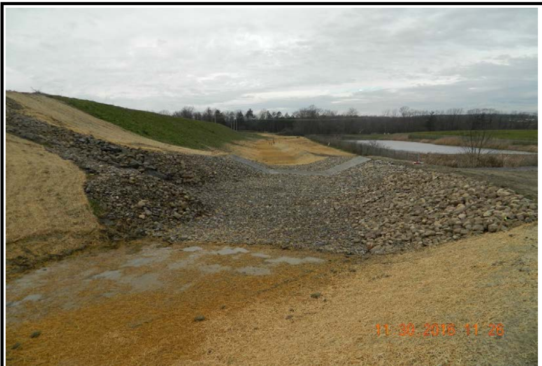
Photo 55: Junction Area, looking west (11/30/16)
