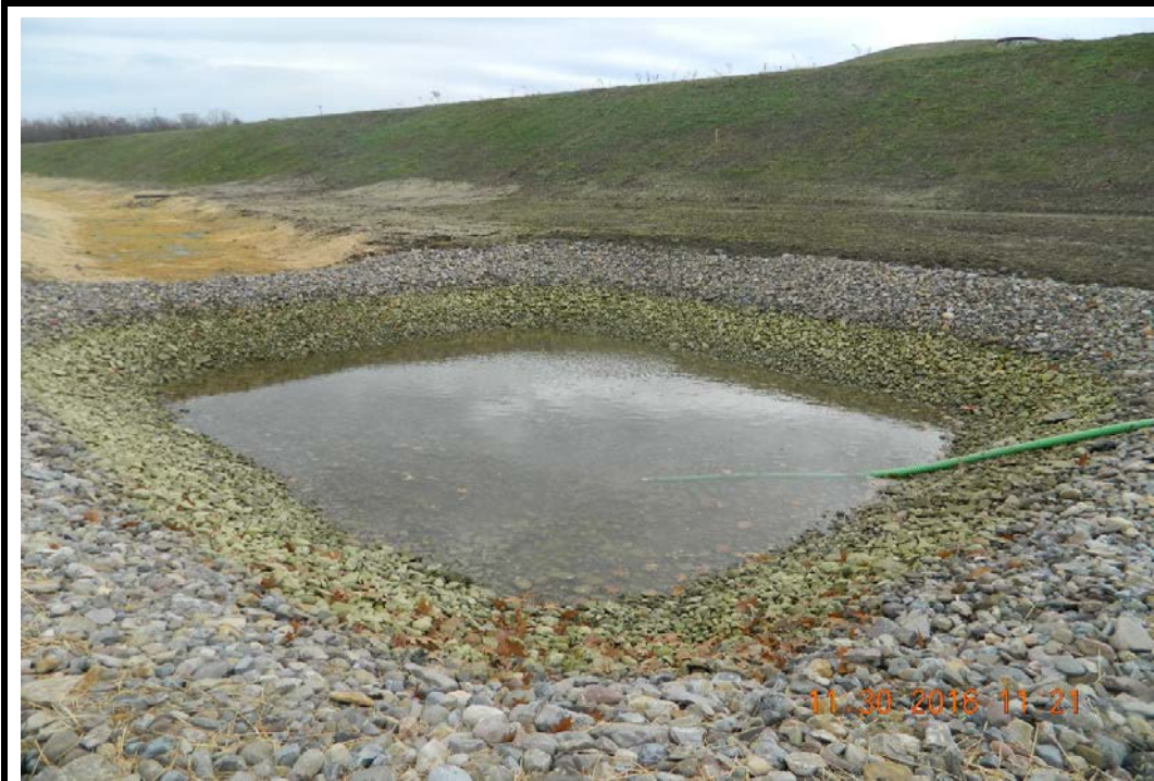
Photo 46: Forebay 1 outlet, looking southeast (11/30/16)
