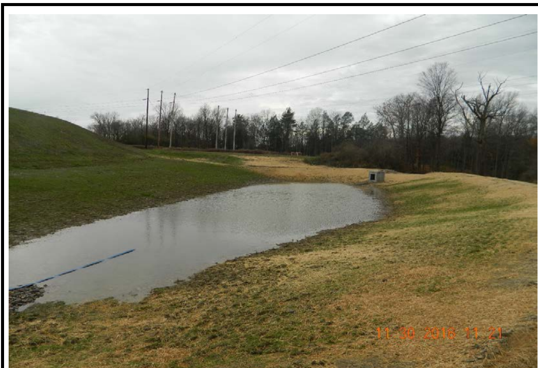
Photo 35: Sediment Basin 1, looking west (11/30/16)
