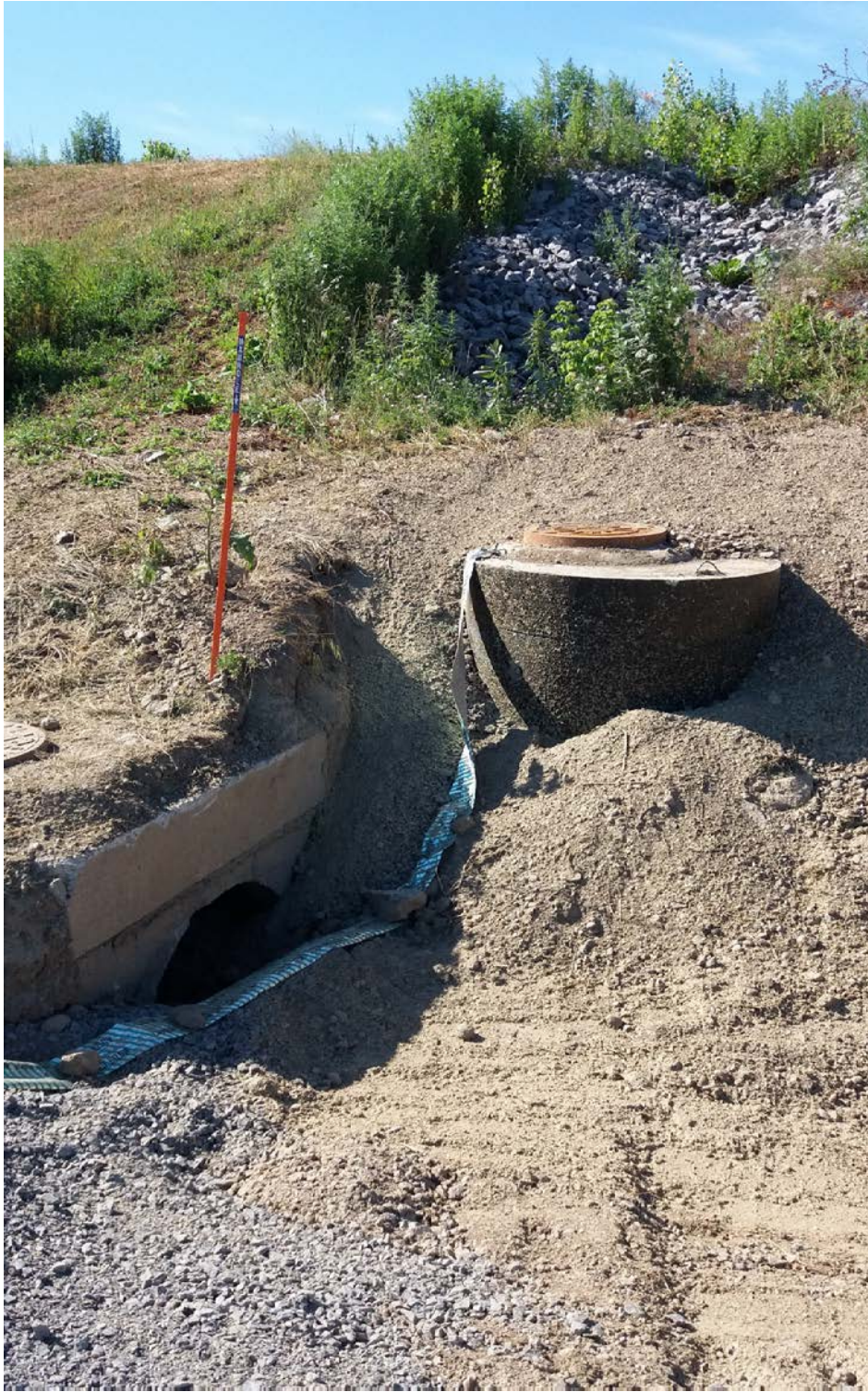
Photo 9 - Final location of MH OADS-3 (6/30/16)
