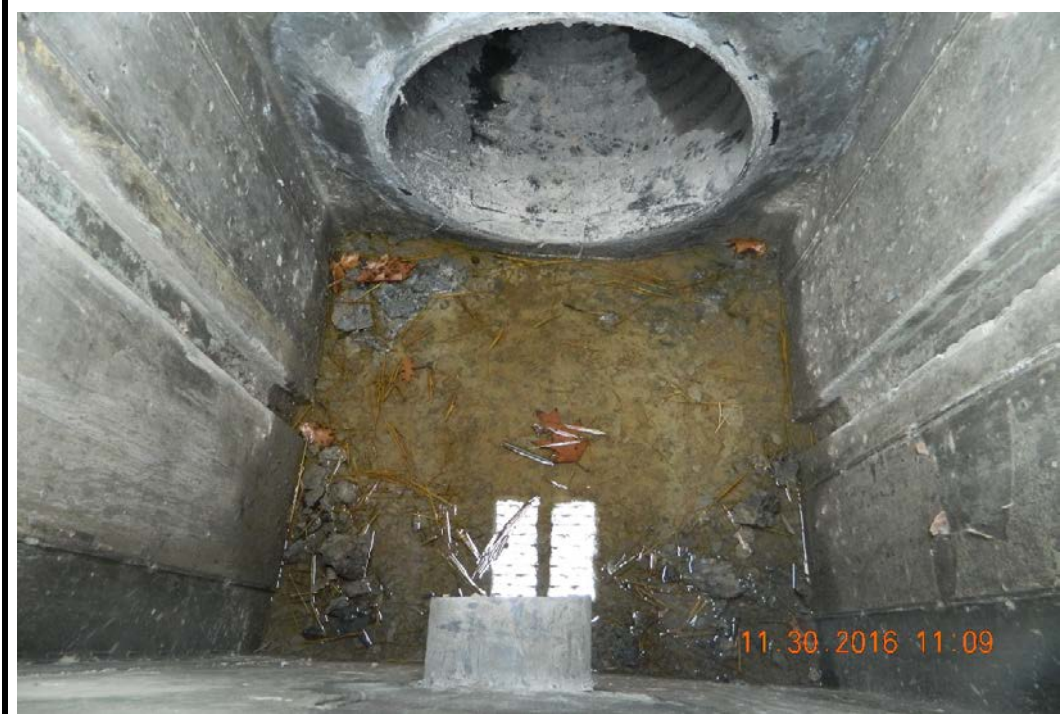
Photo 40: Inside Riser Structure (11/30/16)
