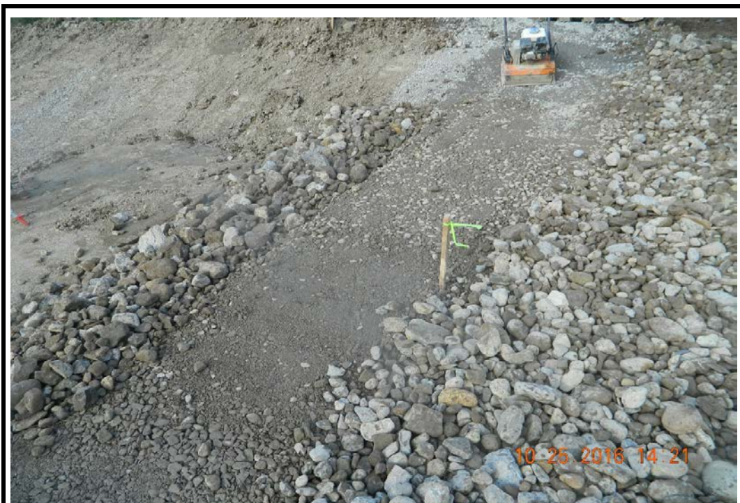
Photo 59: NYSDOT 304-2.01 Type 2 Stone Backfill and adjacent NYSDOT 620-2.02 Light Stone Fill (10/25/16)
