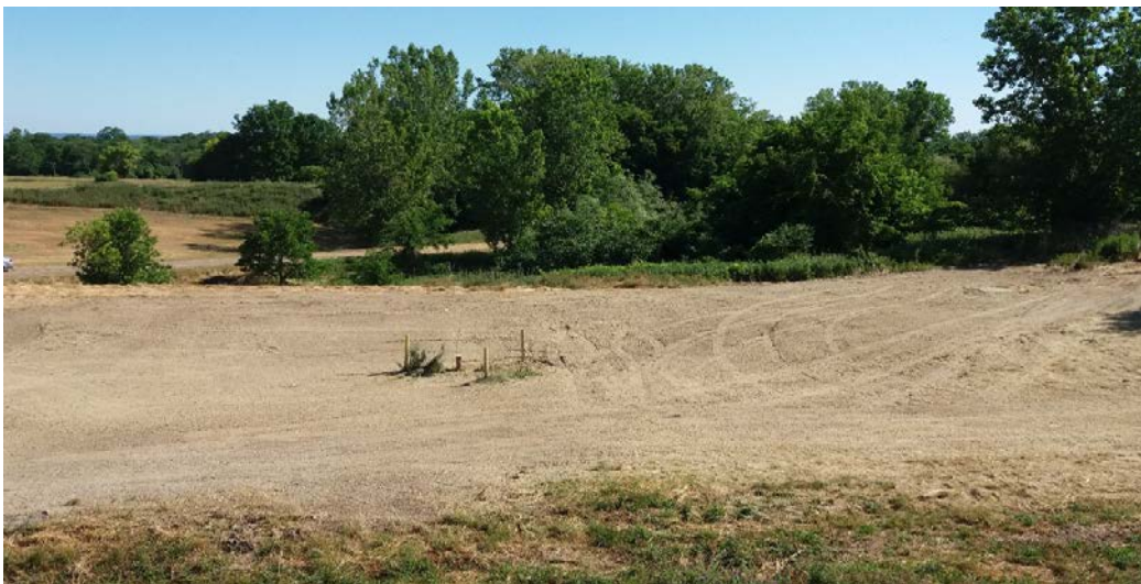
Photo 12 - Interim grading of site (prior to Stormwater Separation Plan) (6/30/16)
