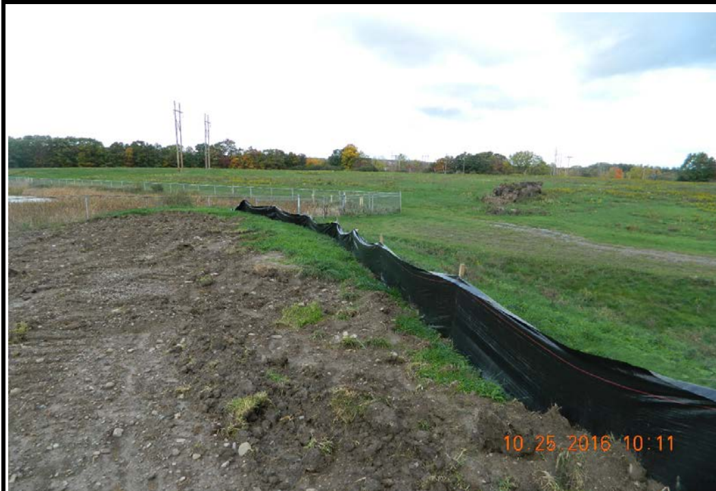
Photo 26: Silt fence installed east of Leachate Pond, looking west (10/25/16)
