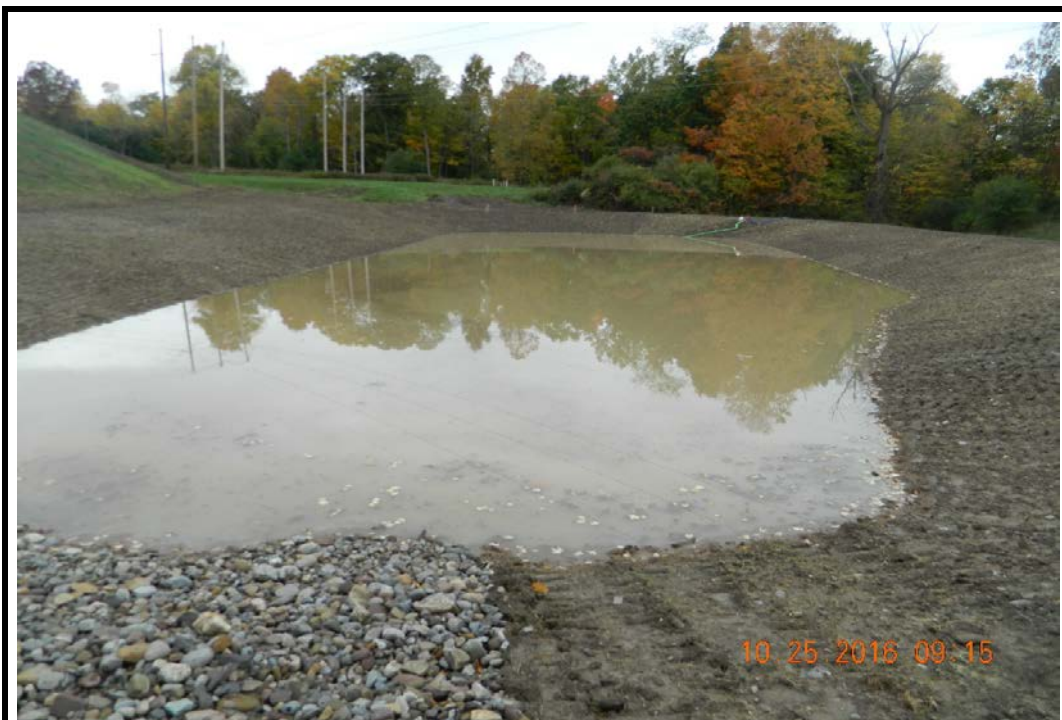
Photo 33: Sediment Basin 1, looking west (10/25/16)
