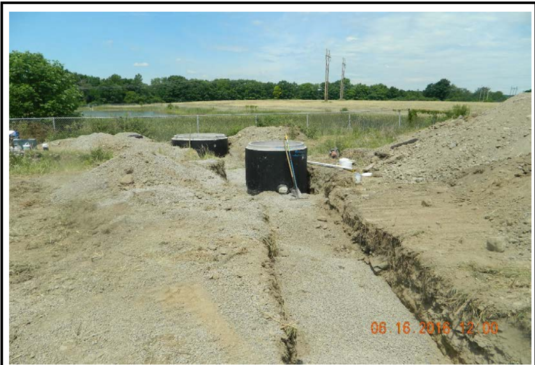
Photo 3 - Installation of Leachate Meter Pit and MH COMMON-1 (6/16/16)
