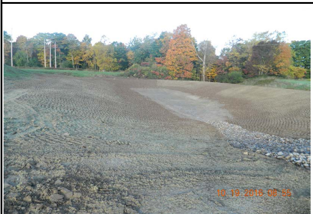
Photo 32: Sediment Basin 1, looking west (10/19/16)
