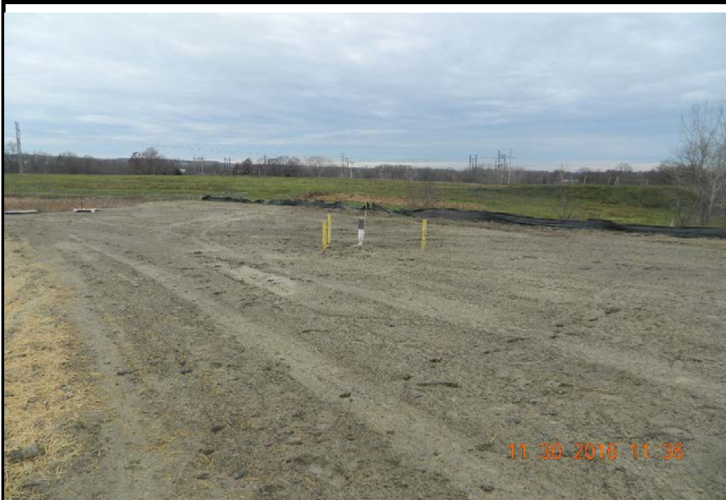
Photo 62: Finished grading north of Junction Area, looking north (11/30/16)
