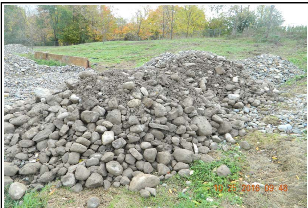
Photo 29: Medium Stone Fill stockpile (10/25/16)
