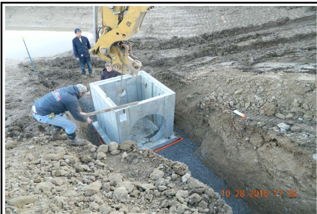
Photo 37: Placing and leveling Riser Structure on bedding, looking southwest (11/8/16)
