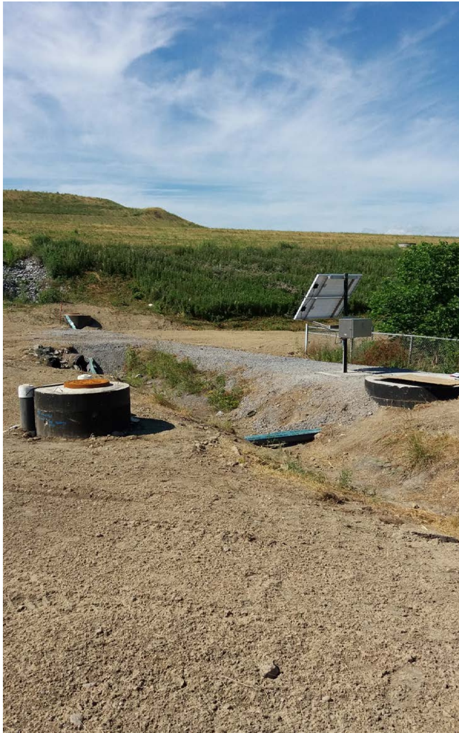
Photo 13 - View of MH COMMON-1 and Leachate Meter Pit (6/30/16)
