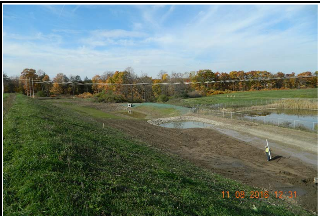
Photo 45: Sediment Basin 1 and Forebay 1, looking northwest (11/8/16)
