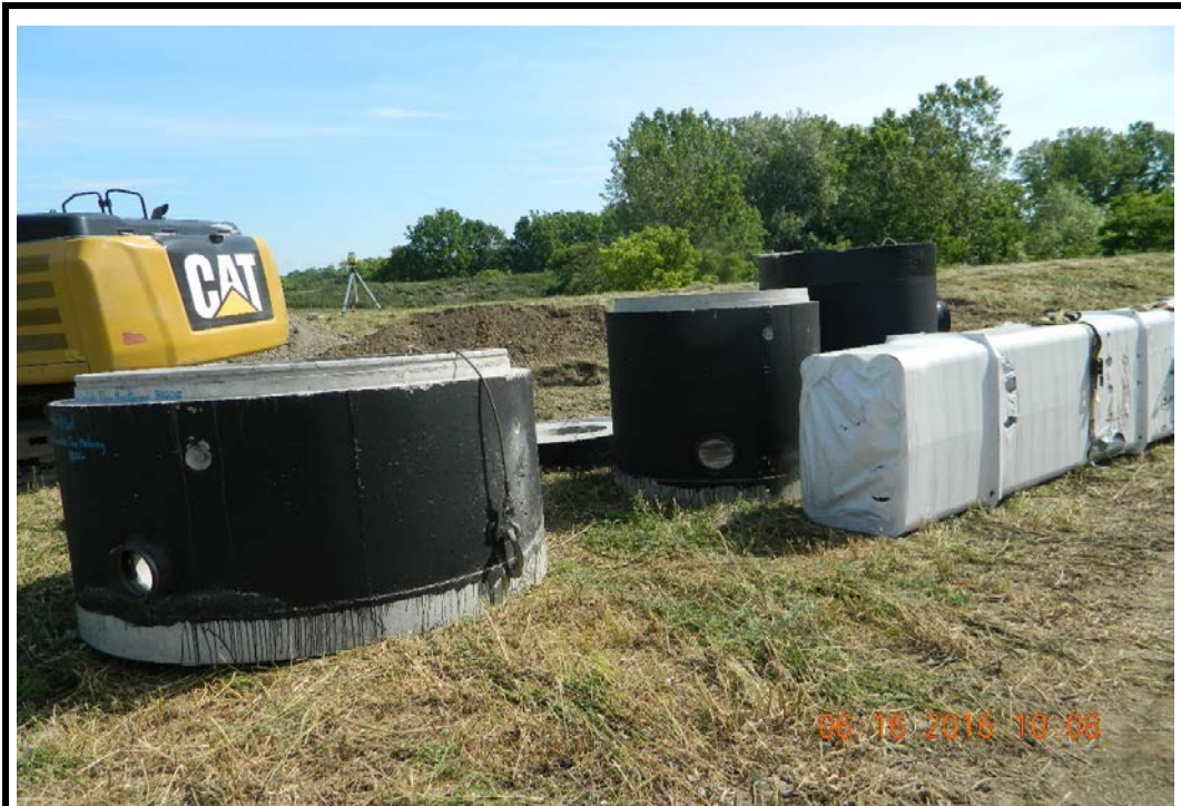
Photo 1 - Manholes prior to installation (6/16/16)
