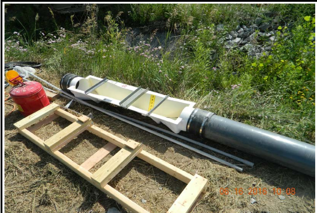
Photo 2 - Flume prior to installation (6/16/16)
