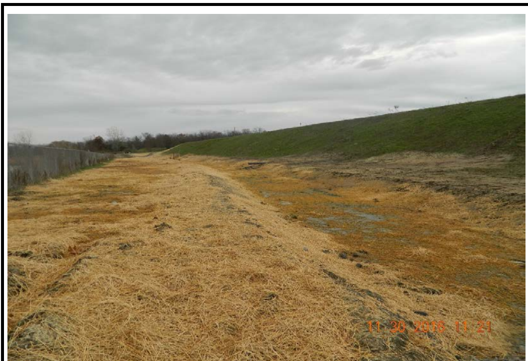
Photo 47: North Channel, looking east (11/30/16)
