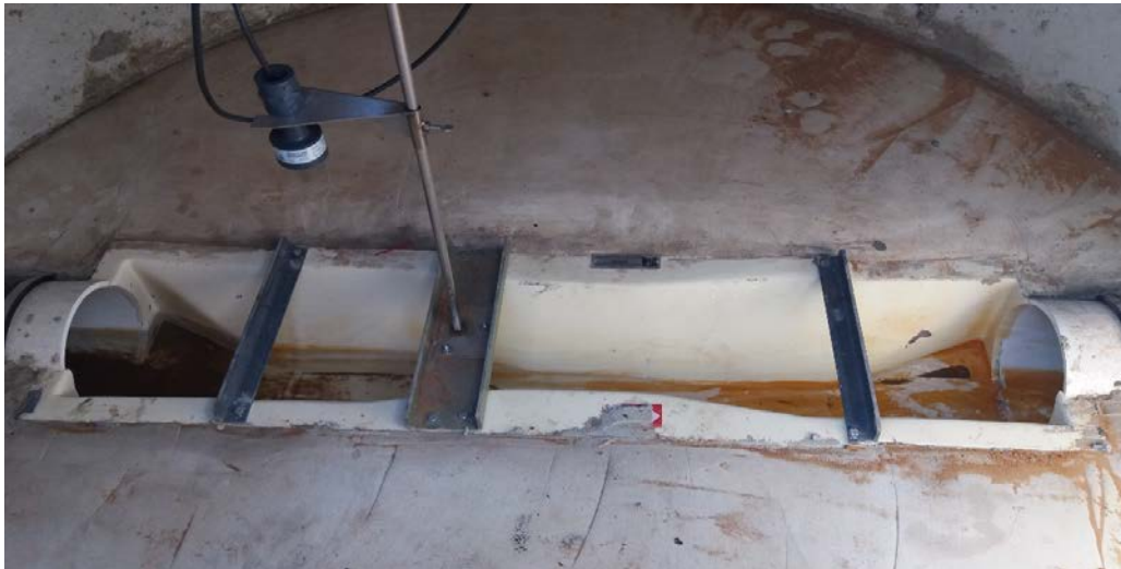
Photo 16: VPC Large 60-degree V Trapezoidal Flume in Meter Pit, with sensor installed (6/30/16)
