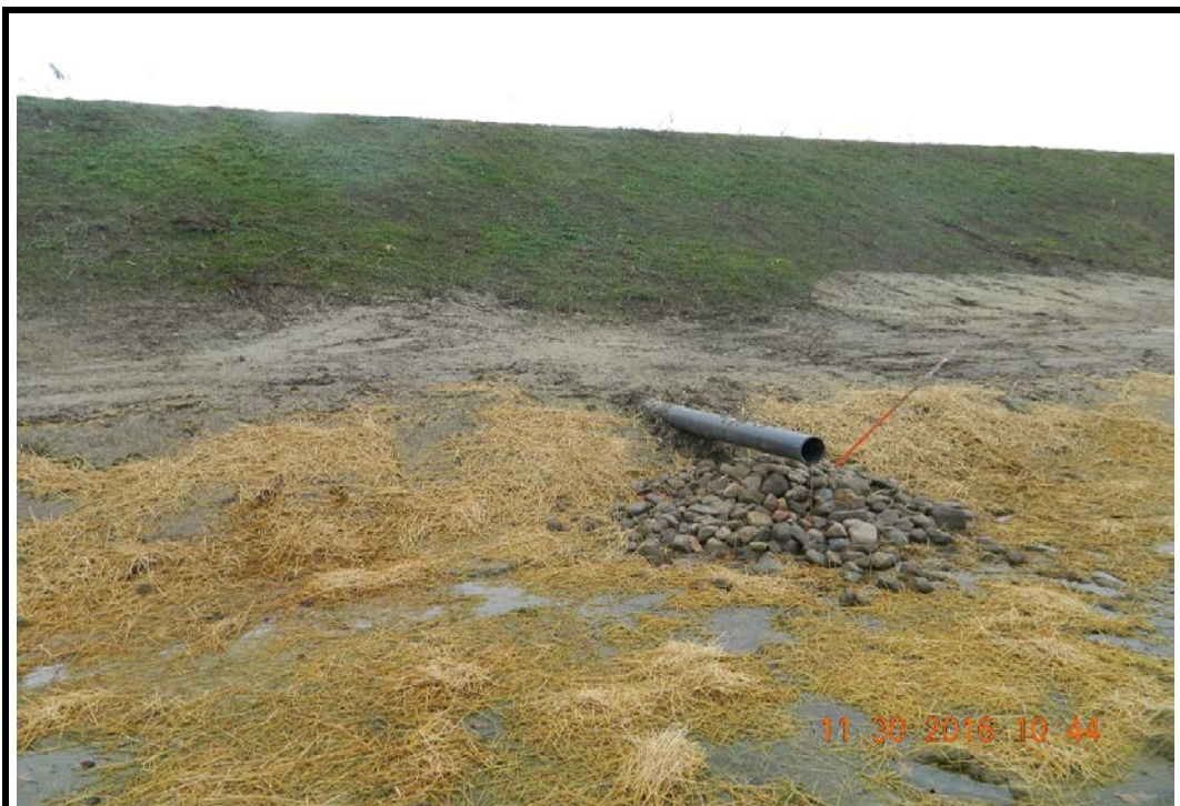
Photo 51: GD-01, looking north (11/30/16)
