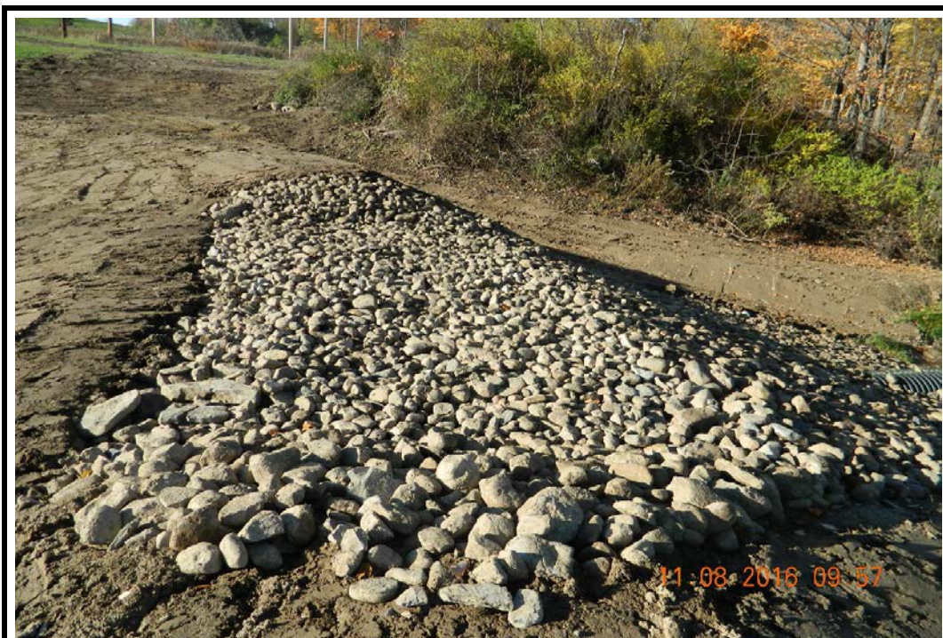
Photo 43: Sediment Basin 1 Emergency Spillway, looking south (11/8/16)
