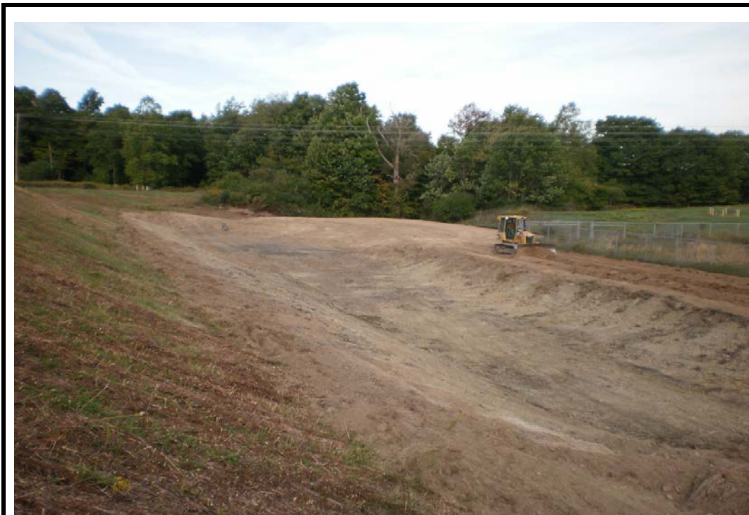
Photo 31: Sediment Basin 1, looking west (9/26/16)
