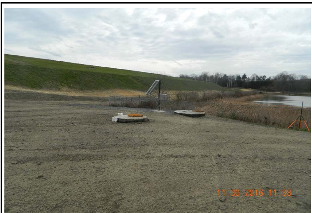
Photo 63: Backfilled concrete lined channel, looking southwest (11/30/16)
