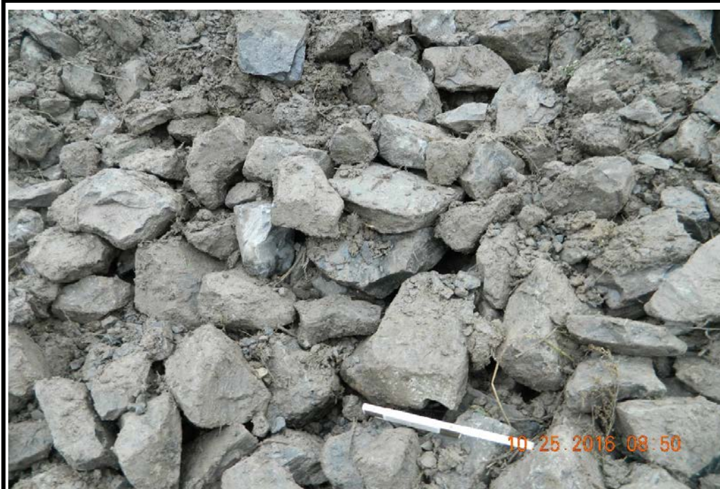
Photo 30: Medium Stone Fill to be reused from downchute (10/25/16)
