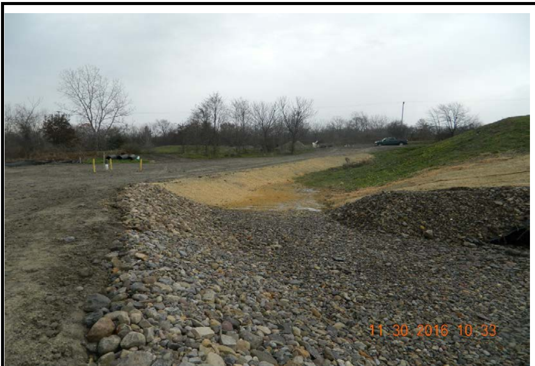
Photo 57: Transition channel east of Junction Area (11/30/16)
