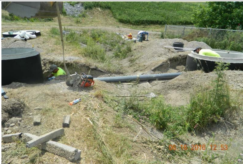
Photo 4 - Installation of pipe between Leachate Meter Pit and MH COMMON-1 (6/16/16)
