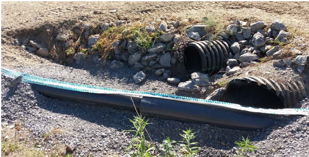
Photo 11 - Eight-inch pipe crossing and termination of 12-inch casing (6/30/16)
