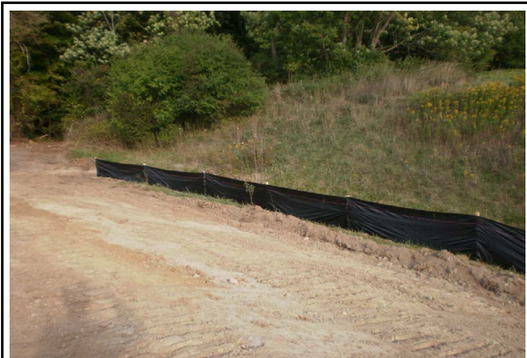
Photo 19: Silt fence installed north of Sediment Basin 1, looking west (9/26/16)
