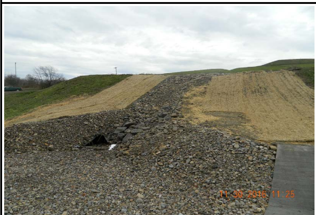
Photo 56: Junction Area, looking north (11/30/16)
