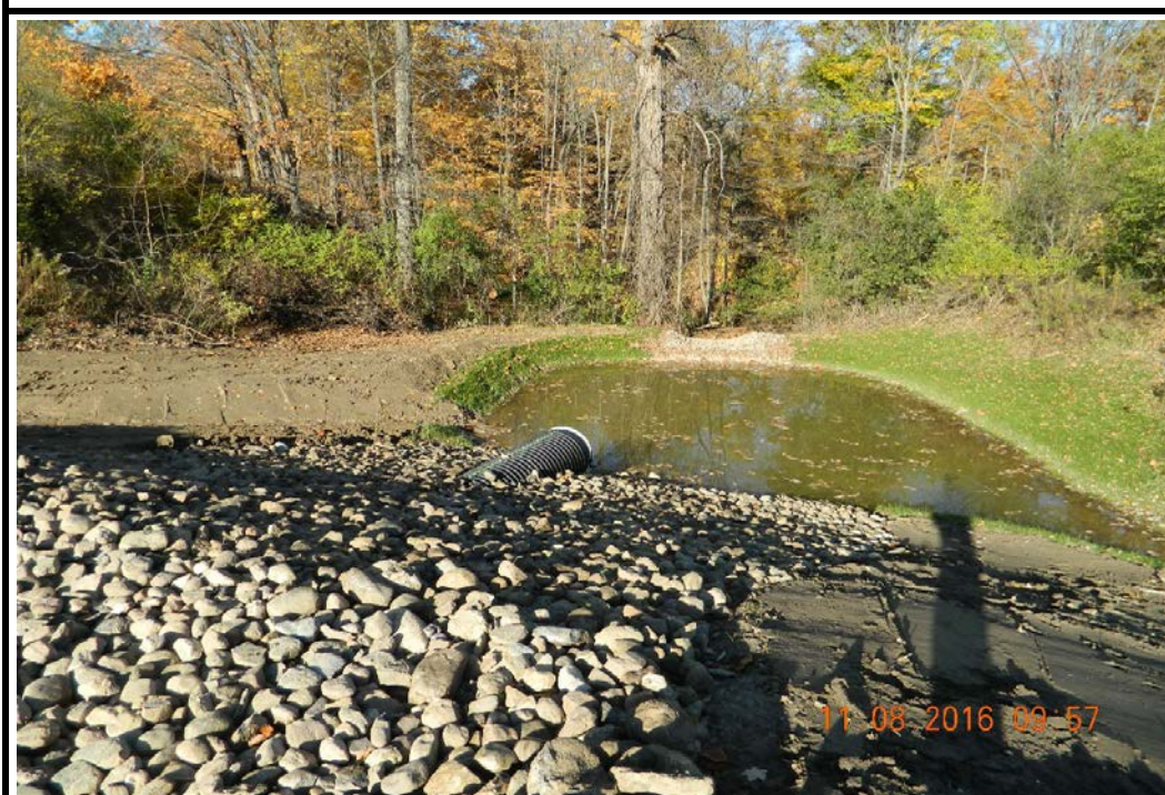
Photo 44: Sediment Basin I Emergency Spillway, looking west (11/8/16)
