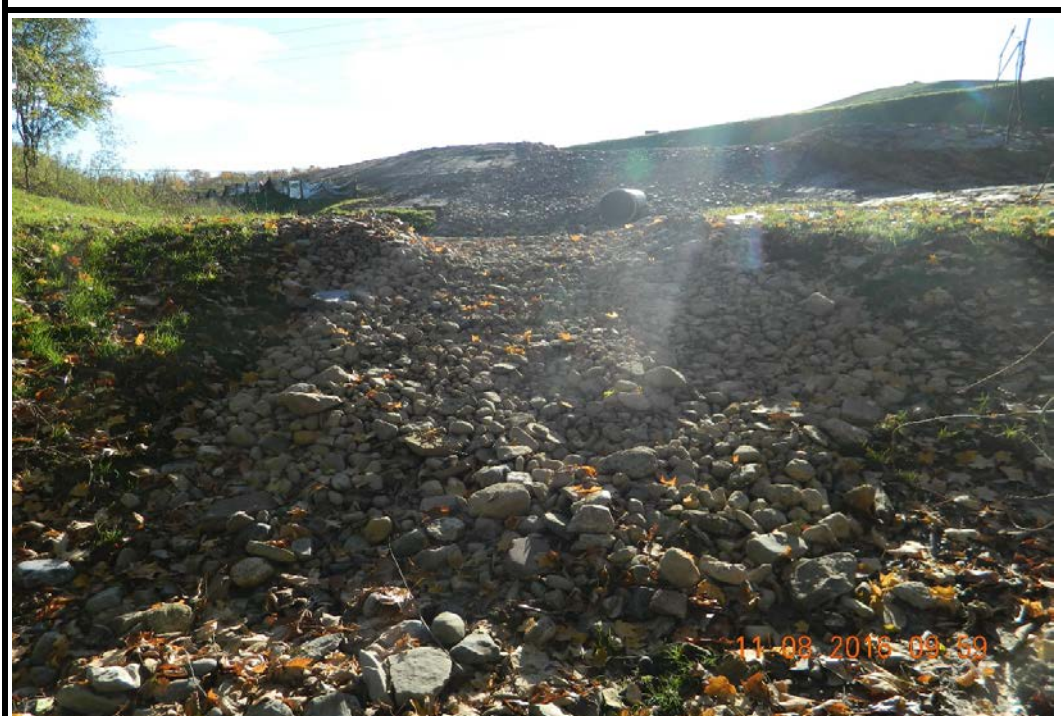
Photo 24: Sediment Trap 1 outlet, looking east (11/8/16)
