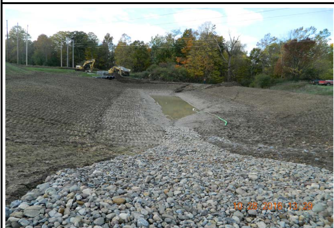
Photo 34: Sediment Basin 1, looking west (10/28/16)
