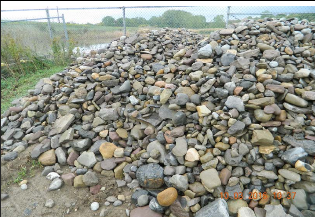
Photo 28: Light Stone Fill stockpile (10/3/16)
