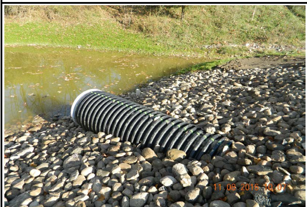
Photo 42: Outlet of 30" Corrugated HDPE Discharge Pipe (11/8/16)
