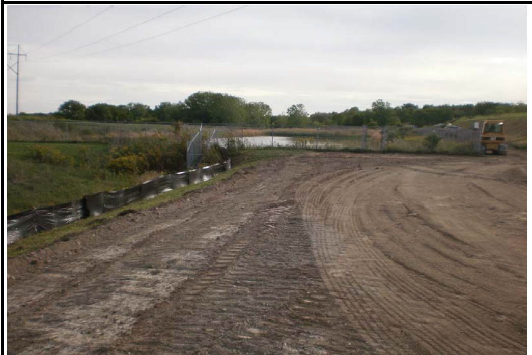
Photo 20: Silt fence installed north of Sediment Basin 1, looking east (9/26/16)
