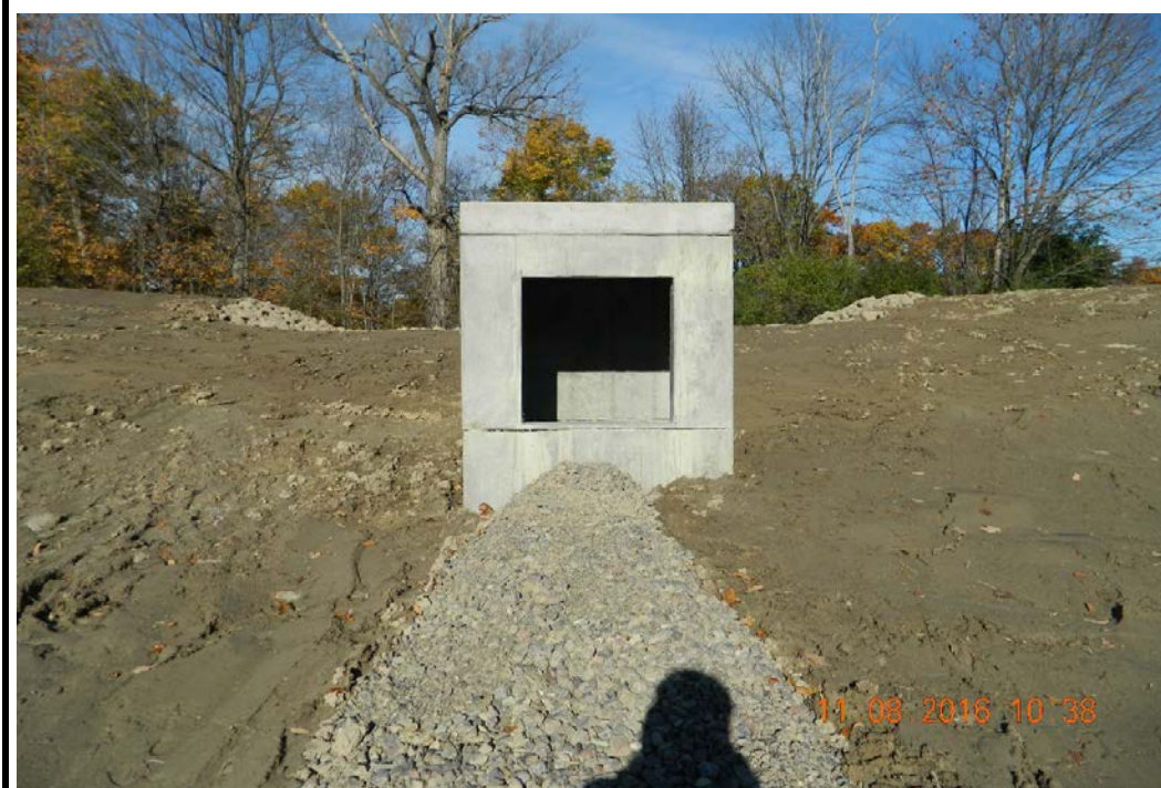
Photo 38: Installed Riser Structure, looking west (11/8/16)
