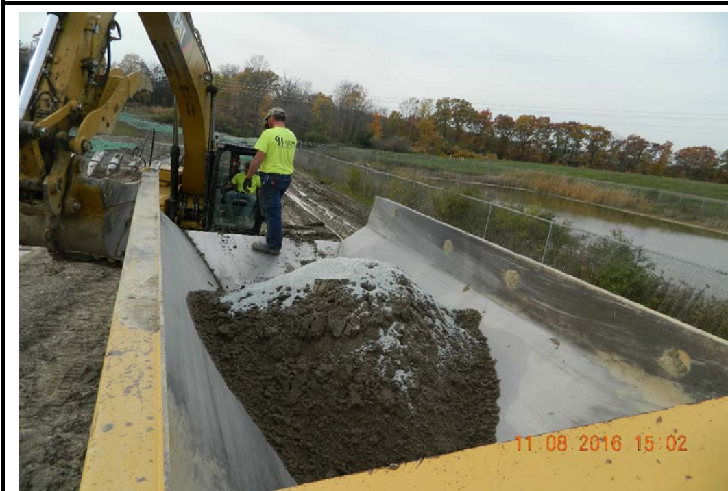
Photo 54: Preparing sand-bentonite mixture (11/8/16)
