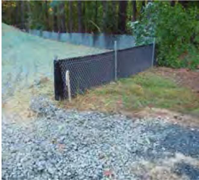
2. Fence Posts (for fabricated units): The length shall be a minimum of 36 inches long. Wood posts will be of sound quality hardwood with a minimum cross sectional area of 3.5 square inches. Steel posts will be standard T and U section weighing not less than 1.00 pound per linear foot. Posts for super silt fence shall be standard chain link fence posts.
